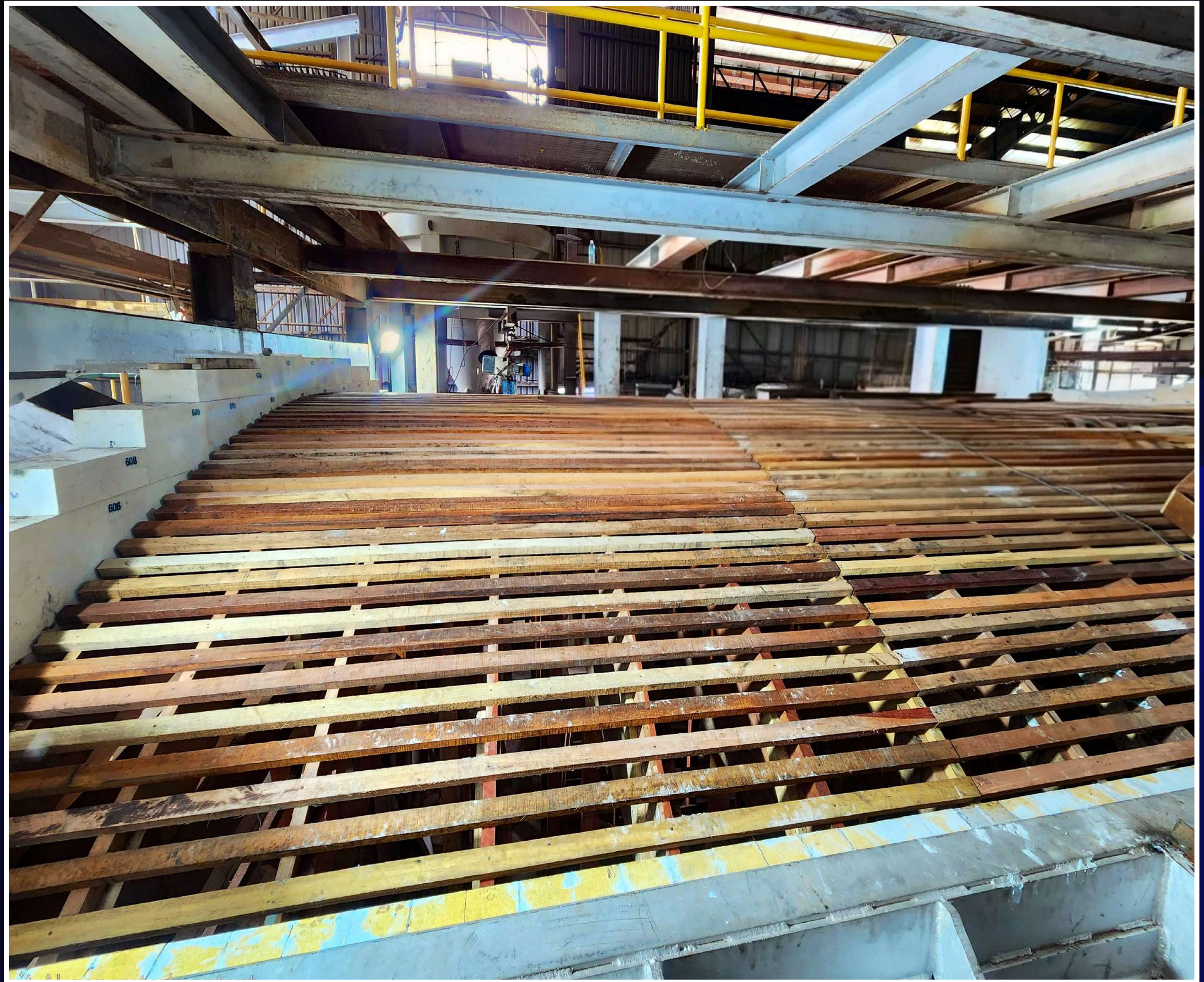
Wooden Centerings – Furnace Crown
