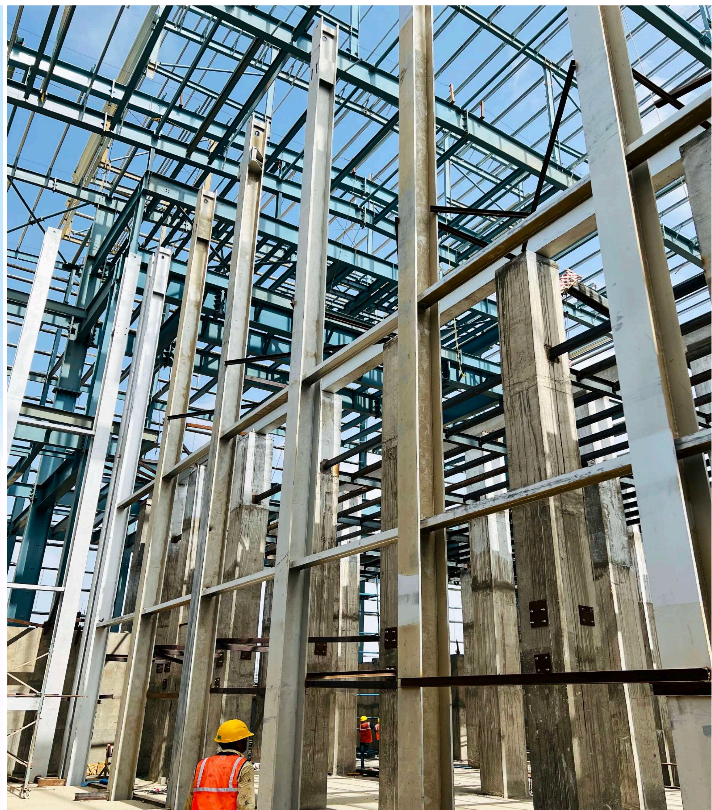
Erection of Steel: Regenerators – LHS & RHS
