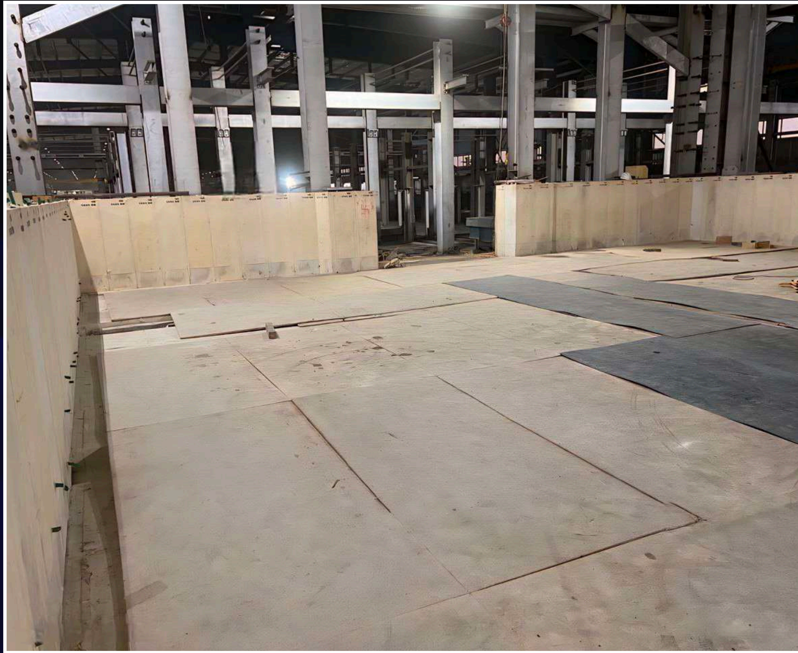
Refractory Installation – Melting Tank & Refiner
