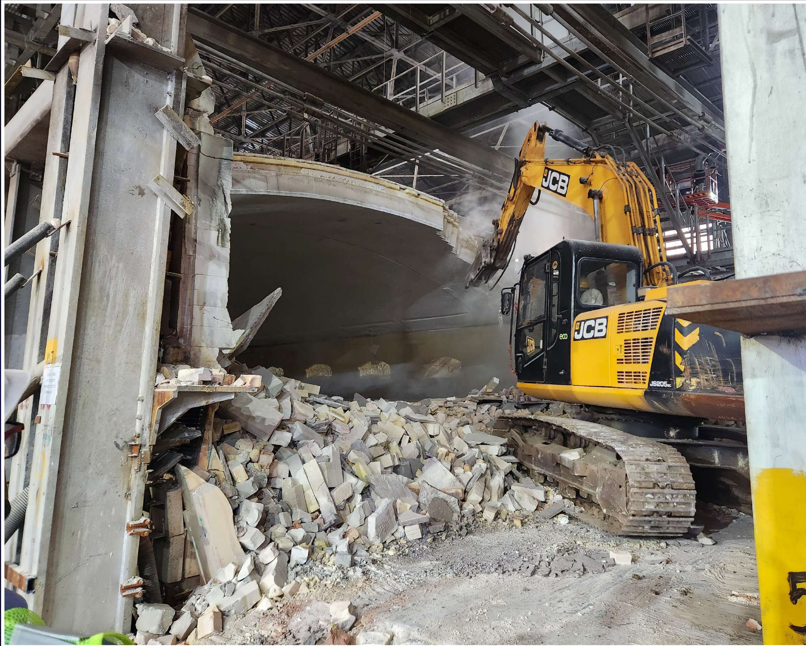
Demolition of Furnace
