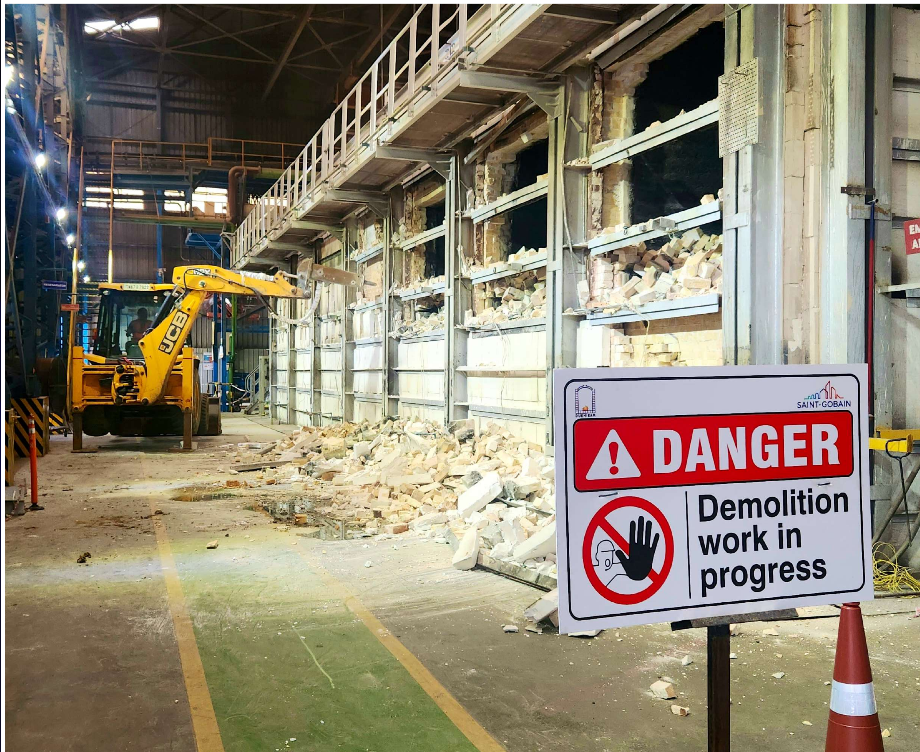
Demolition of Regenerators
